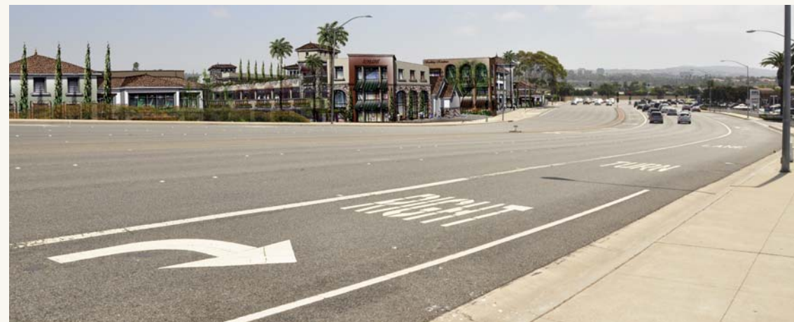
View from Bridge along East Coast Highway
